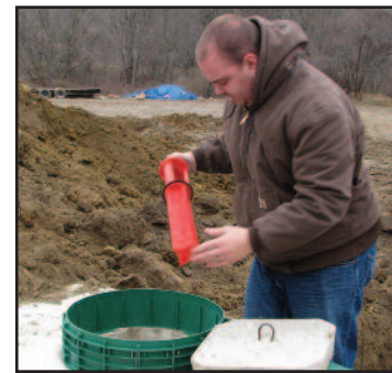
Kyle Shackle, RS, inspects a septic system at a new home construction site to make sure it has been installed correctly.
